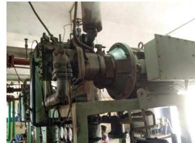
Figure 5: Ammonia Compressor installed
